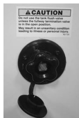
Tank Flush Inlet
