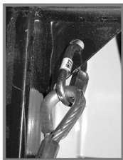
Quick Link cable hook-up at top of the door frame
